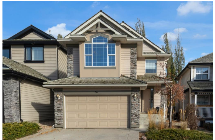
26 Springbank Rise SW, Calgary, AB
